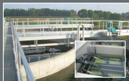
Agristo (Potato processing) Membrane Bio-Actor Water Reuse
