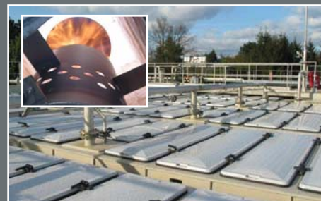
Alken Maes (Brewery) Anaerobic Bio-Actor Green Energy
